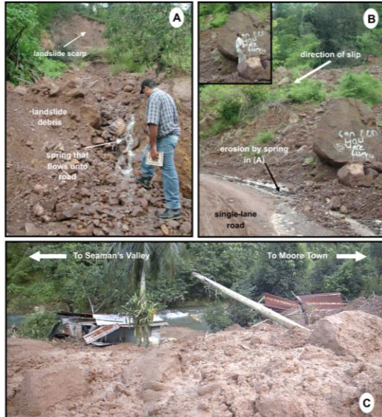
Figure 1. Rainfall-induced landslide (November 2005) at London along the Seamans Valley to Moore Town Road, Rio Grande Valley, in weathered volcanic rock and shale. Classified as a rock slump–debris/earth flow. Damage included blocked road, four houses obliterated along with personal effects of occupants, light pole toppled and water main severed. (A) View up-slope of landslide (left-hand side facing the landslide). The scarp is the source area for the material. Perched groundwater emerging from the landslide body results in the spring. (B) View along road looking towards Moore Town (right-hand side facing the landslide). The spring in (A) has eroded a channel in the road. Unstable debris continued blocking the road as the material settled. The partly stable boulder in the foreground threatened road users. The inset shows the size of the boulder compared to the size of a man. (C) Remains of houses destroyed by the landslide (toe-area of landslide). Three of the obliterated houses were at this location; only two are visible. Note the toppled electrical pole. [S. Bhalai, Dec. 2005 and R. Green, Nov. 30, 2006].
