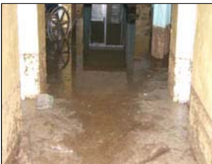
Main hall at the emergency department of Jimaní's Hospital
