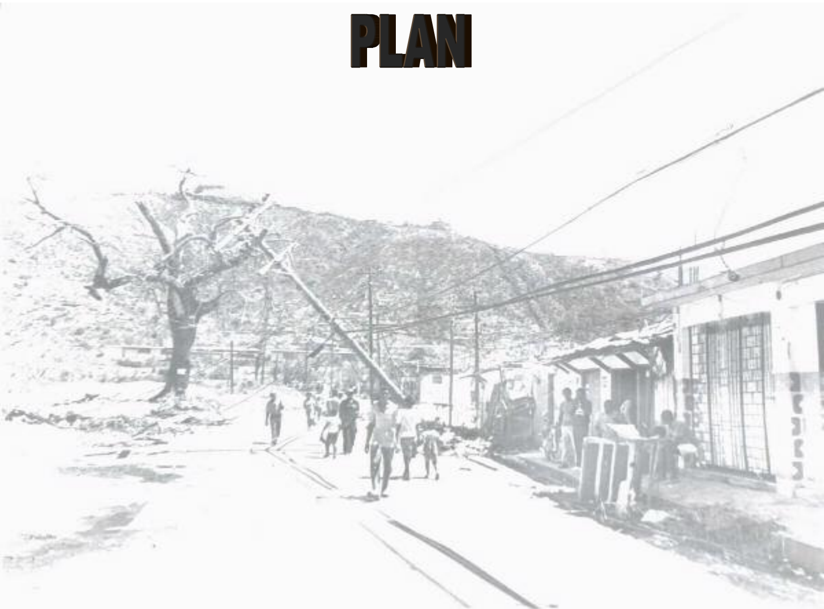
Damage caused by Hurricane Gilbert, 1988.
